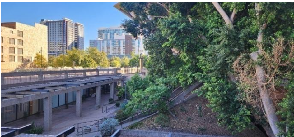
City of Tempe, AZ, USA. Trees on the City Hall and Surrounding
